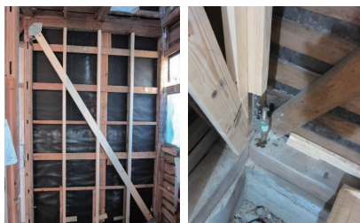
Reinforcement of walls
